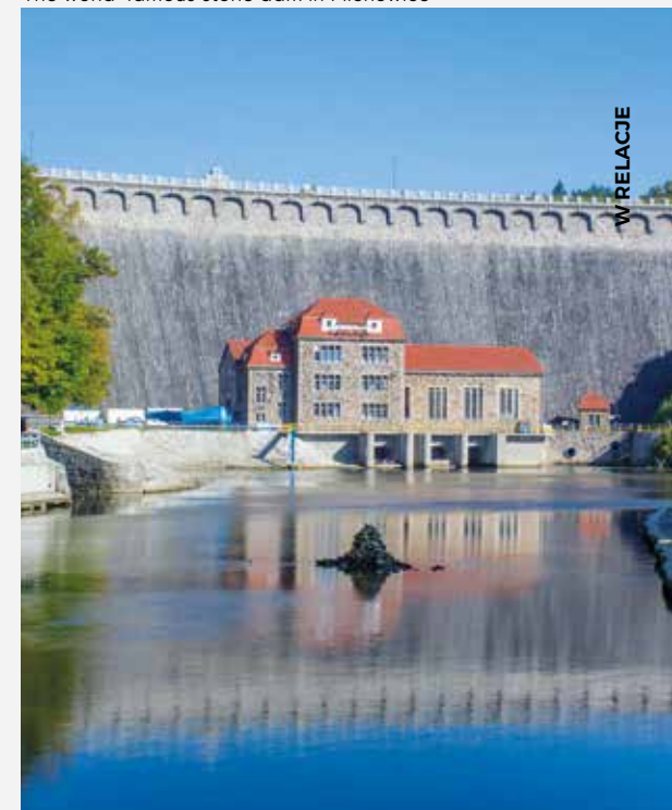
Kamienna zapora w Pilchowicach / The world-famous stone dam in Pilchowice
